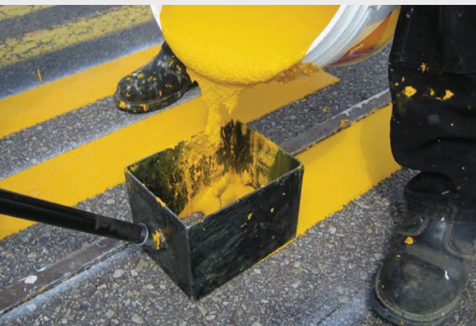
Transverse marking application
