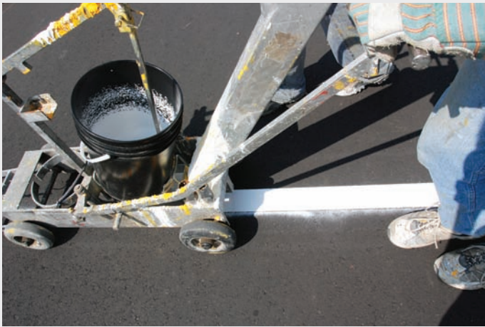
Cold Plastic applied using a walk-behind applicator
