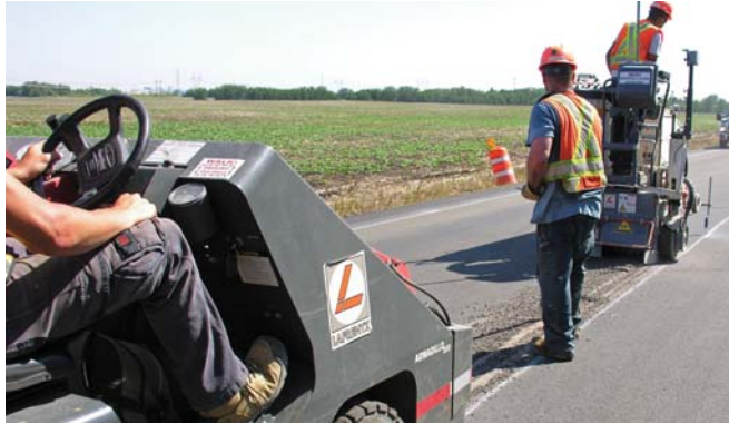
Milling the groove
