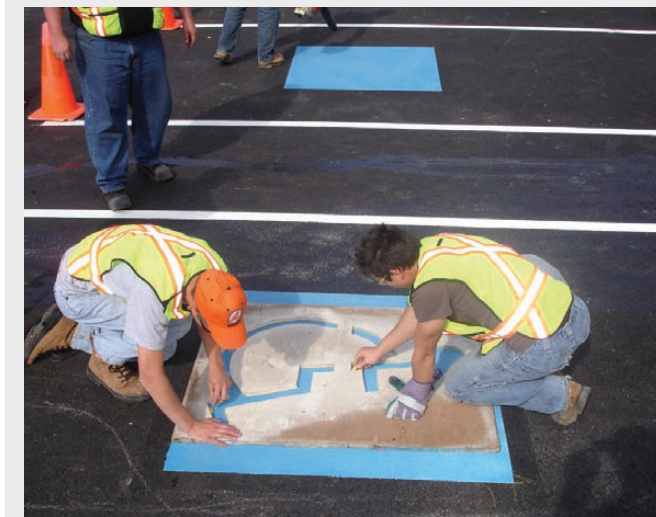
STEP 5: Installing complicated symbols
