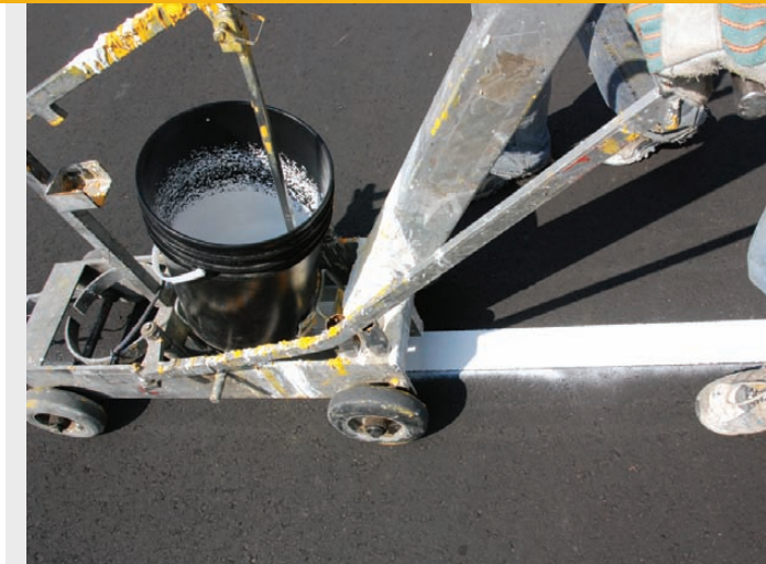
STEP 4: Longitudinal line application
