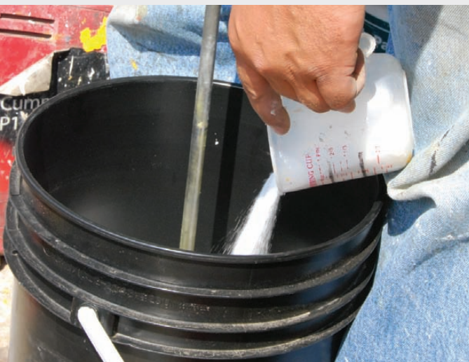
STEP 2: Adding the catalyst
