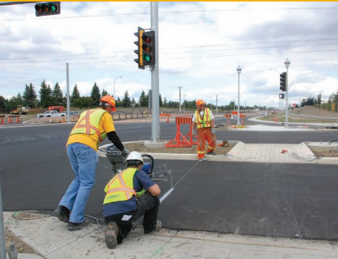
STEP 1: Pre-marking the lines
