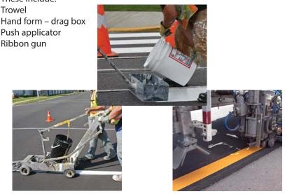
Extrusion material can be applied on the roadway surface or in a groove or filling the groove and over banding.
