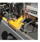
The surface should be free of debris and dust, perfectly clean and absolutely dry. At a minimum sweeping and air blast of the surface is required.
