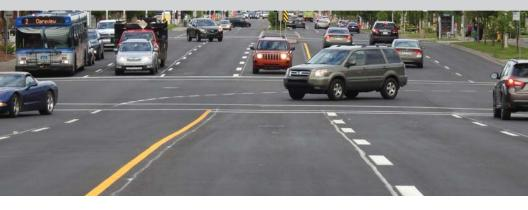
Thermoplastic pavement marking materials utilize heat to generate a bond to the asphalt cement in the pavement surface. These materials are manufactured to be applied onto the pavement in molten form with glass spheres mixed in and also dropped on the material immediately after it is applied.
