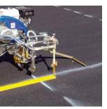
Liquid material should be sprayed at the specified thickness from edge to edge across the entire marking. Immediately after the liquid material self-levels glass beads should be applied evenly across the marking. There should be enough glass bead to saturate the liquid and leave some loose beads on the surface. Once the marking has cured excess glass beads should be removed as they present a safety hazard.
